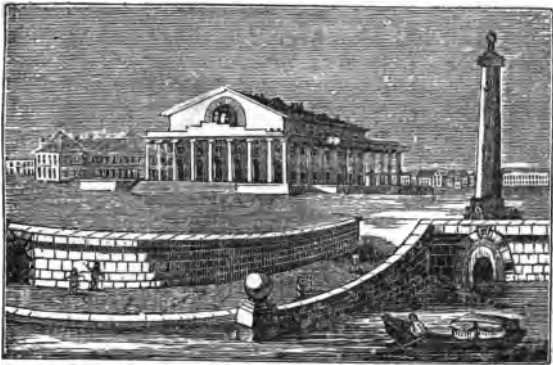
View of the Exchange, St. Petersburg.
